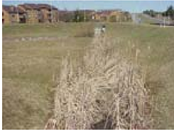
Figure M4.6: Vegetation establishment where the inflow channel slope is inadequate to drain properly.
