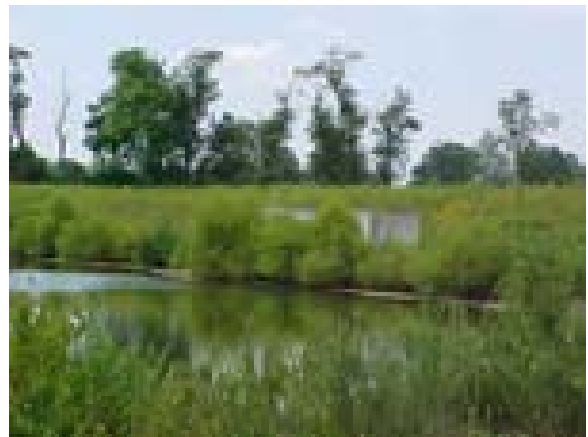
Figure 1.9: Excessive vegetative growth obscures riser
