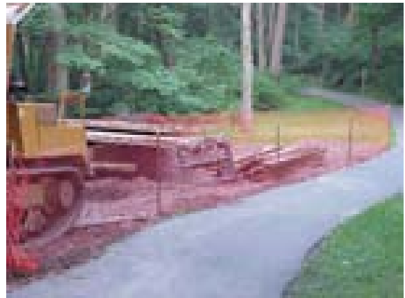
Figure M6.5: Paved access road.
