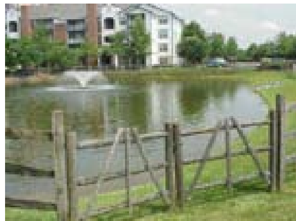
Figure M7.2: Surface aerator / fountain.
