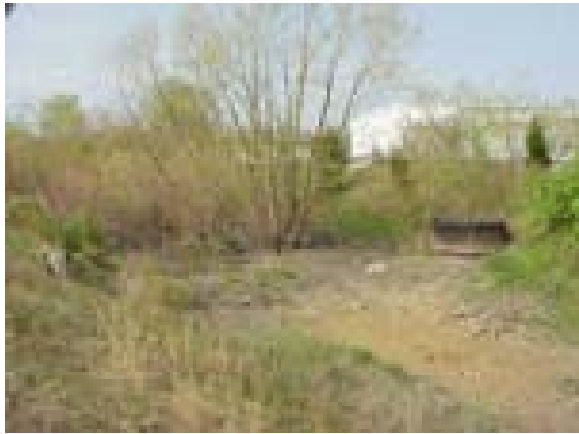
Figure 1.10: Sediment accumulation in a dry pond
